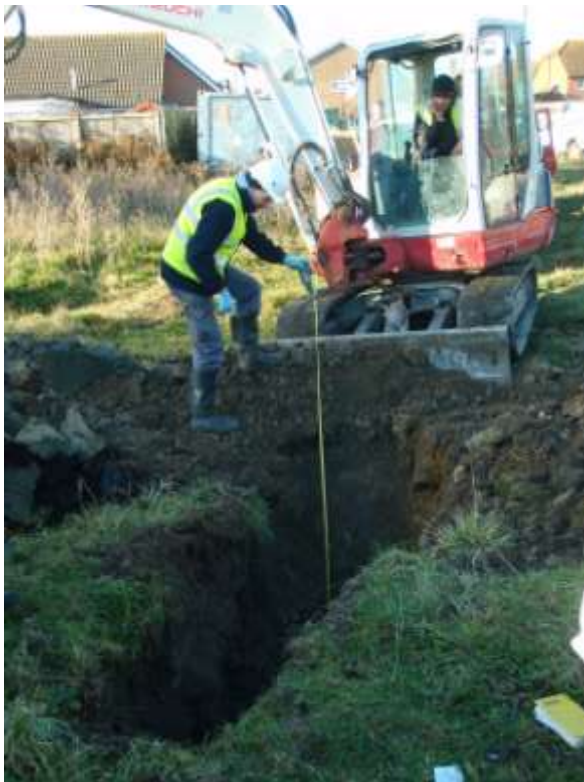
Plate 3. View of site soil investigations (looking NNW)
