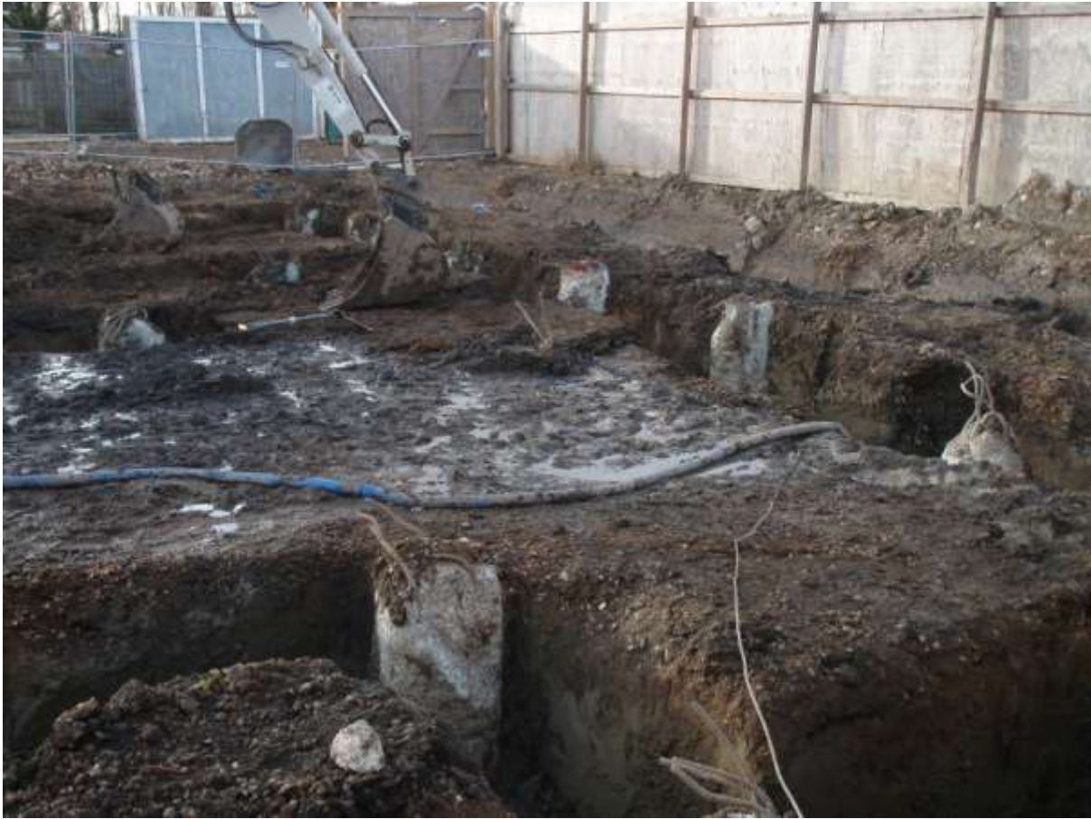
Plate 4. View of site trenching in 2019 (looking W)
