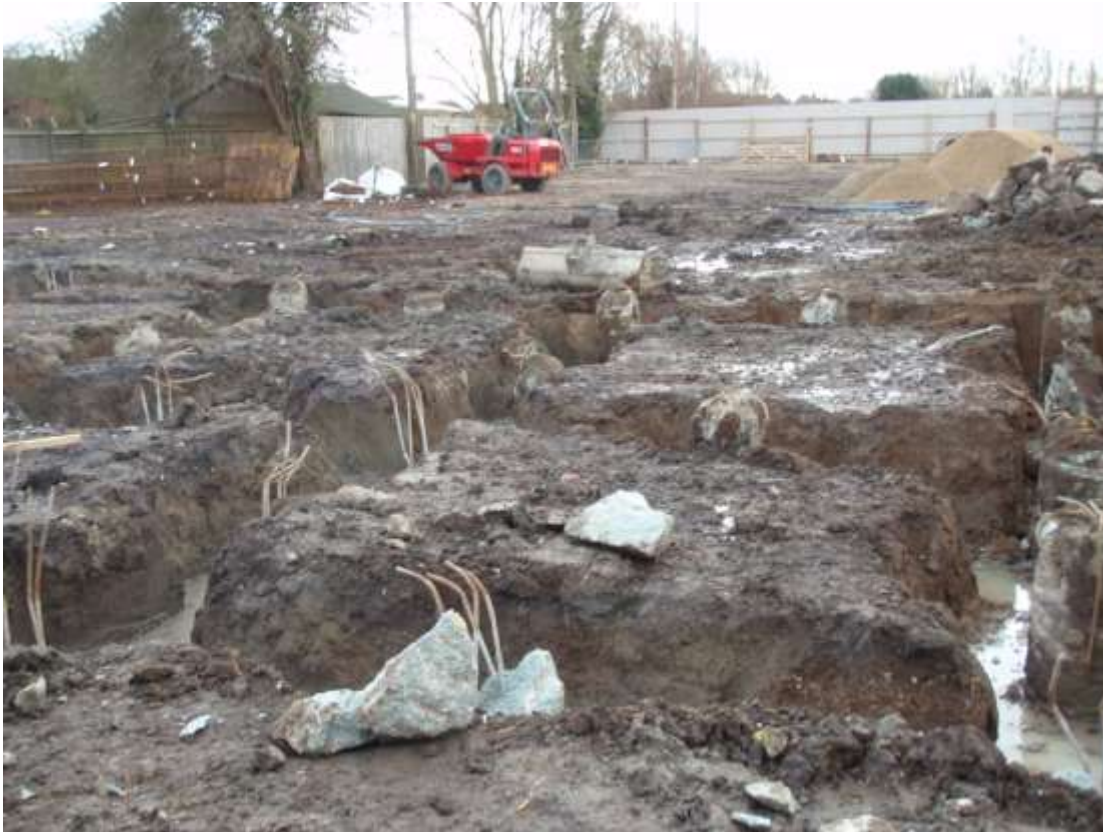
Plate 6. View of the trenches (looking SE)
