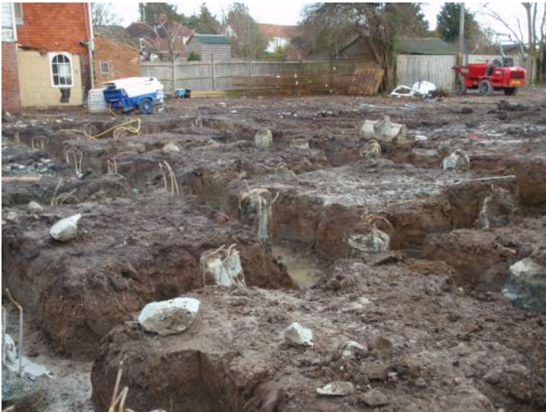
Plate 7. View of the trenches (looking west)
